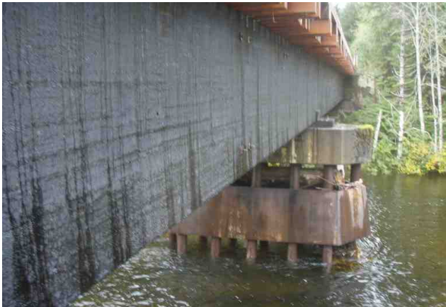
Figure 1-9: Span 1 girder 1 upstream face.
