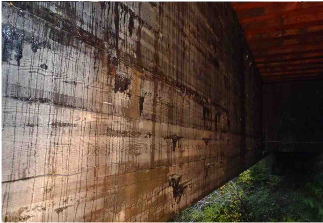
Figure 1-14: Span 2 girder 3 upstream face near pier. (AE2329, AE2341, AE2328)
