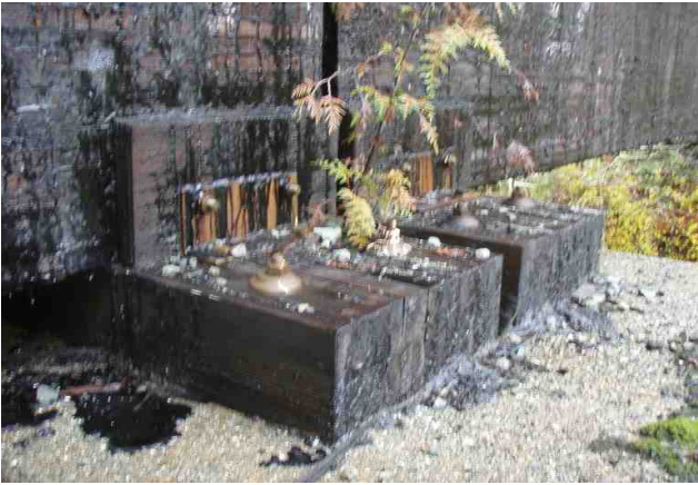
Figure 1-23: Timber sills on pier.
