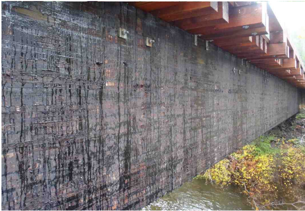
Figure 1-13: Span 1 girder 4 downstream face.
