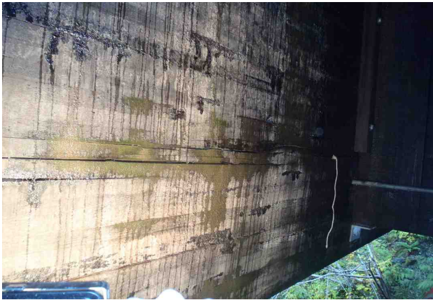
Figure 1-16: Span 2 girder 3 upstream face near woods end.
