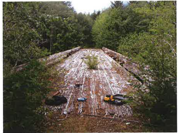
Photo 2 - Typical Condition of Bridge Deck
