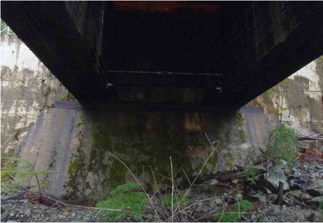
Figure 1-21: Woods end abutment.
