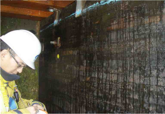
Figure 1-19: Span 2 girder 4 downstream face; end check at woods end.
