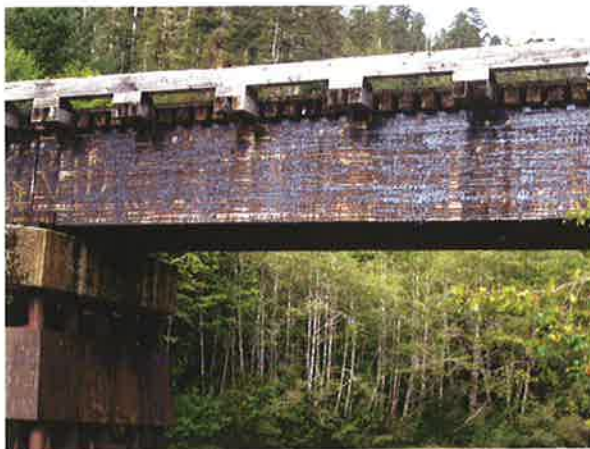
Photo 3 - Typical Condition of Exterior Girder
