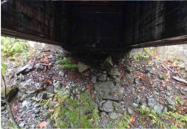
Figure 1-20: Camp end abutment.
