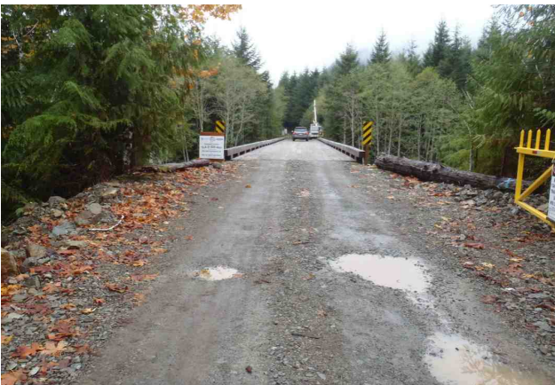
Figure 1-3: Looking towards woods end.
