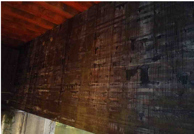
Figure 1-11: Span 1 girder 2 downstream face.
