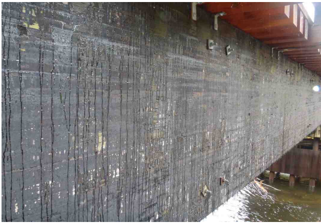
Figure 1-17: Span 2 girder 4 downstream face.
